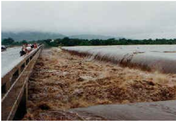
Dam Wall, Komatipoort [Photo: TSB]
